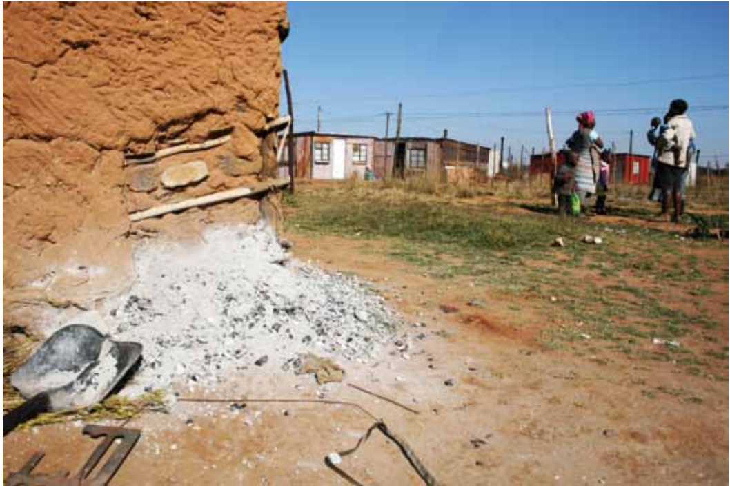
Top: This house in Arbor (Highveld) is crumbling as a result of blasting coming from the coal mine bordering it.
